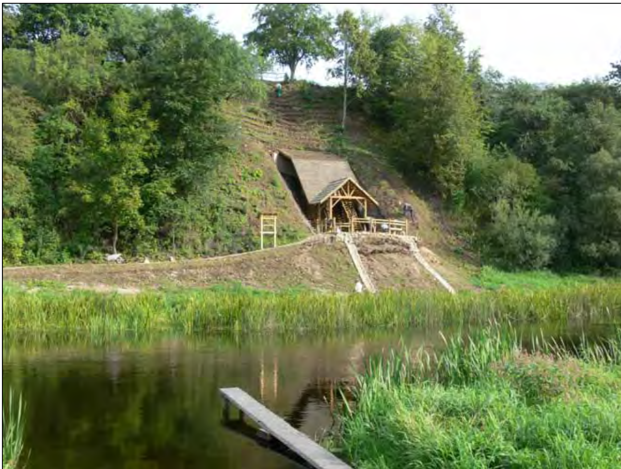
Visiting facility in the Jurassic outcrop in Papilė. The exposure is protected by a shelter, and this is the first of its kind in Lithuania.
