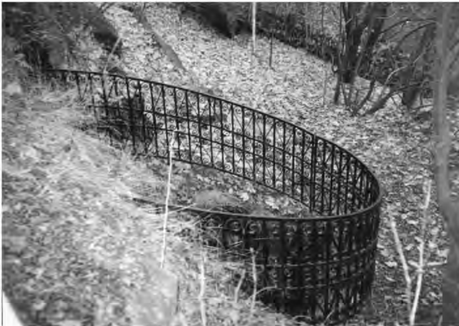
The fence erected around the pot-hole protecting people falling into the pothole
