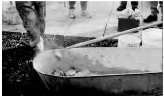
Demonstration of quicklime for use as mortar in restoration, by Scottish Lime. Photo: Sylvia Smith-Meyer
